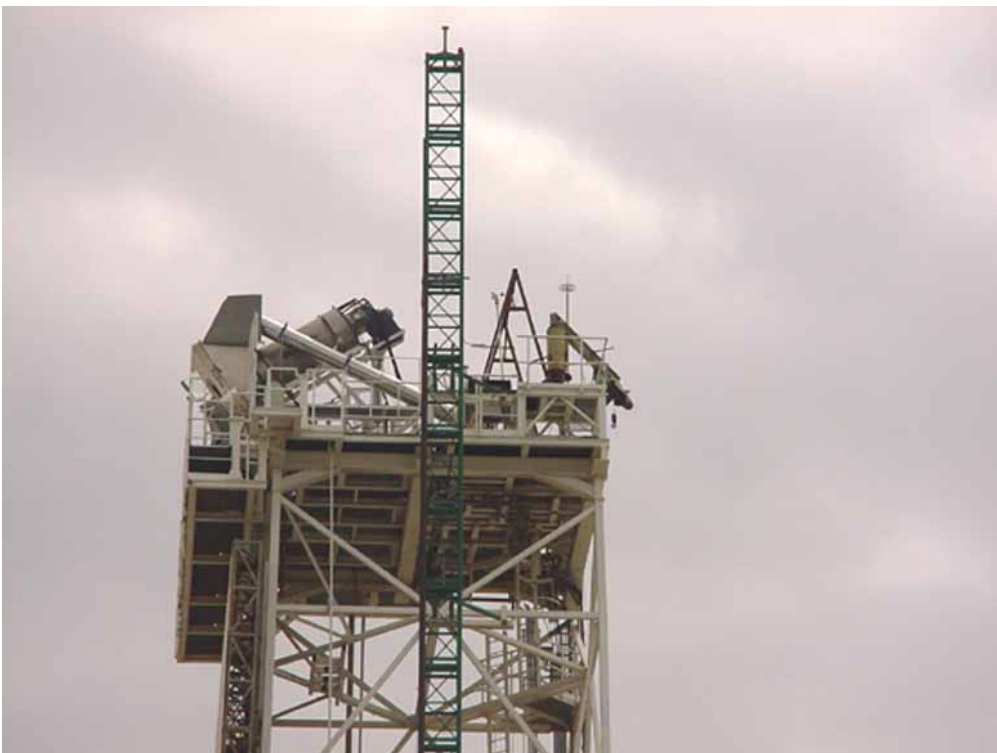
HitRec2 being tested April 2001 with air return piping
