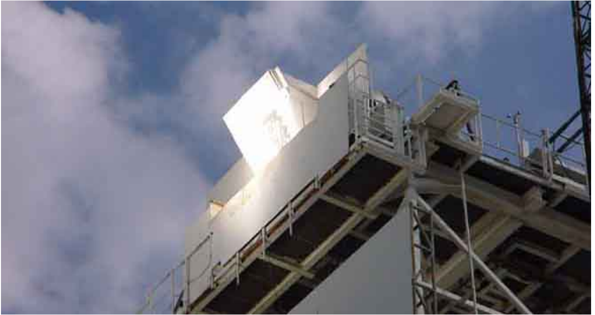
The rectangular shaped HitRec2 system tested fall 2000 with no air-return system
