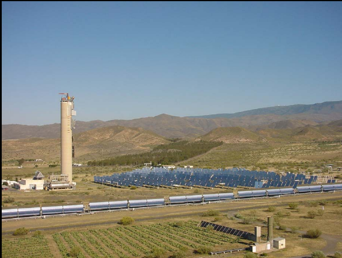
Stobbe Tech & DLR Solar Thermal Power Plant Technology
