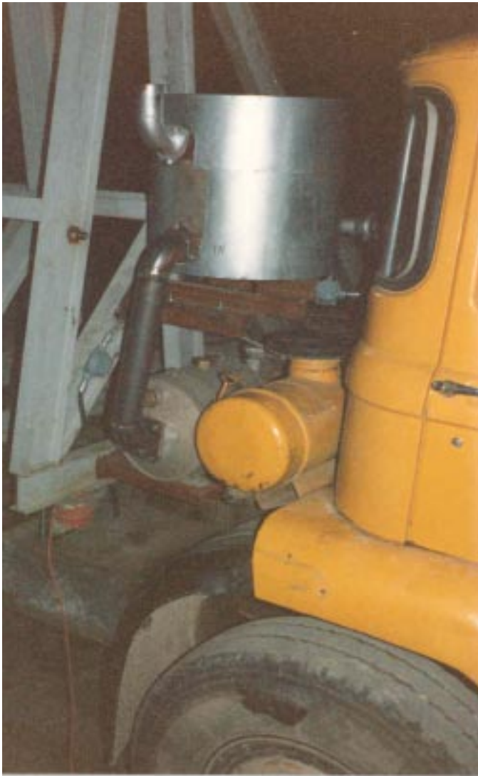
First practical trials in Danmark with Diesel Partikel Filter, on a truck at Tinglev Beton elementfabrik in 1988 performed by the entertainer!
